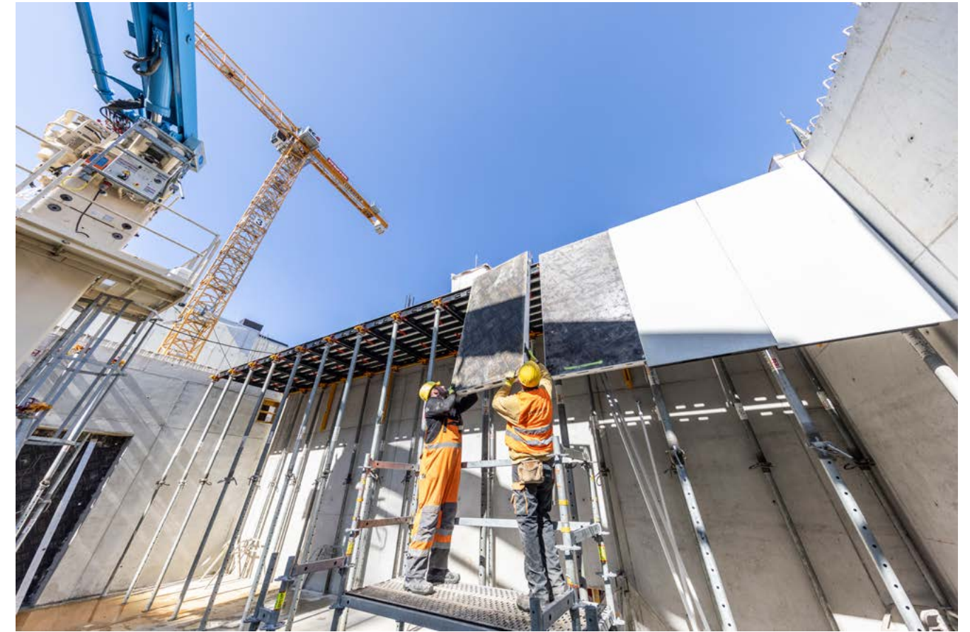
Even high slabs exceeding 3.80 m can be formed from the level below with PERI system components. The compatibility of the aluminium and polymer components enables you to optimally adapt them to your construction site requirements.
