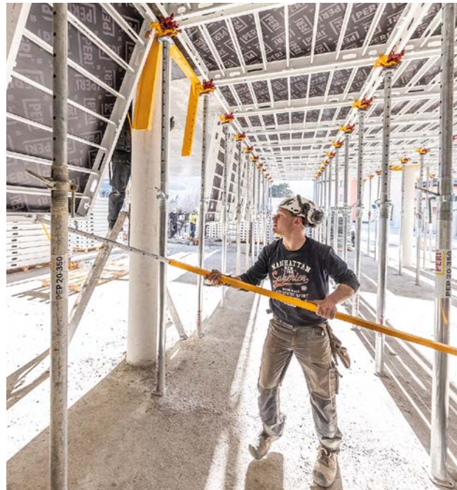
With the shuttering aid you can safely form room heights of at least 3.80 m.
